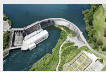
Karāpiro 101MW 515GWh (1946)
