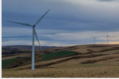
Mahinerangi 36MW 100GWh (2011)
