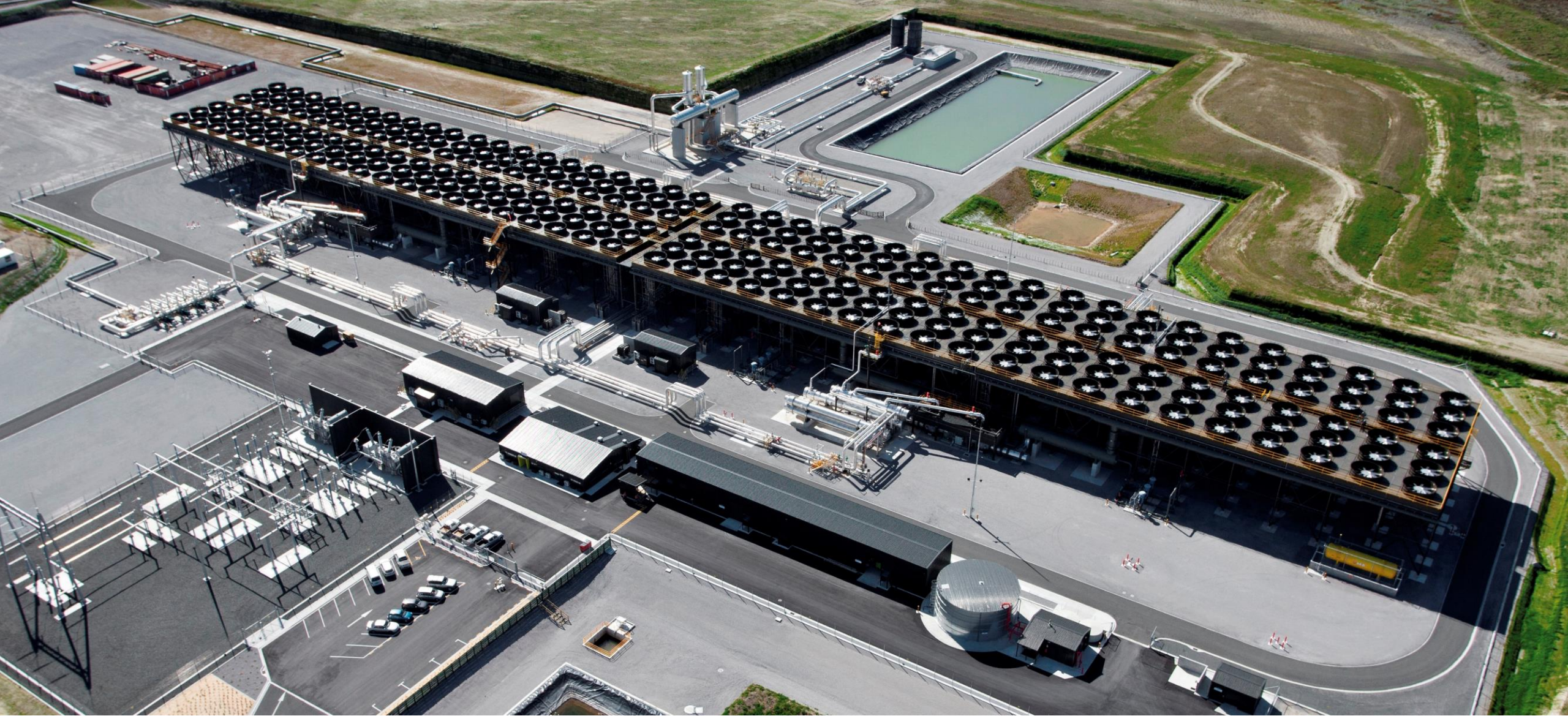
Ngātamariki power station
